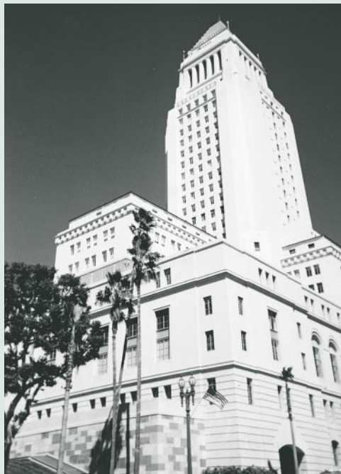
Los Angeles City Hall, dedicated April 26, 1928. Seismic retrofitting and restoration of this historic city landmark was completed in fall 2001. Photo: Jeffrey Levin.
