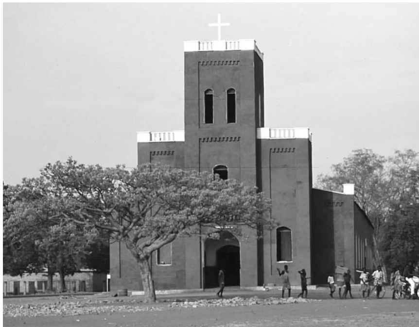
Exterior and interior views of Our Lady of the Seven Sorrows Cathedral, Navrongo, Ghana. Getty funding is supporting comprehensive conservation planning for this last remaining cathedral in Ghana constructed with earthen materials. Photo (exterior): © CRATERre-EAG. Photo (interior): © CRATERre-EAG/T. Joffroy.
