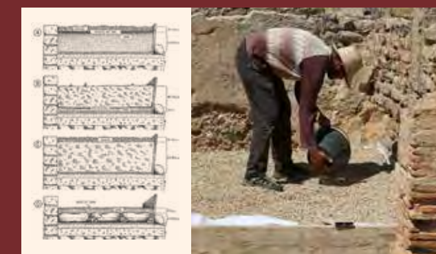
Section drawings of mosaic reburial techniques using different materials (left), a recent reburial in progress (right). Many of the mosaics currently exposed to the elements are located in areas that are not generally visited by tourists or are just easily accessible. The majority of these pavements will be reburied and then returned to their long-term preservation and protection. Reburial is a critical component in planning for the future conservation of Bulla Regia, taking into account the site's available human and financial resources, which need to be carefully managed.
