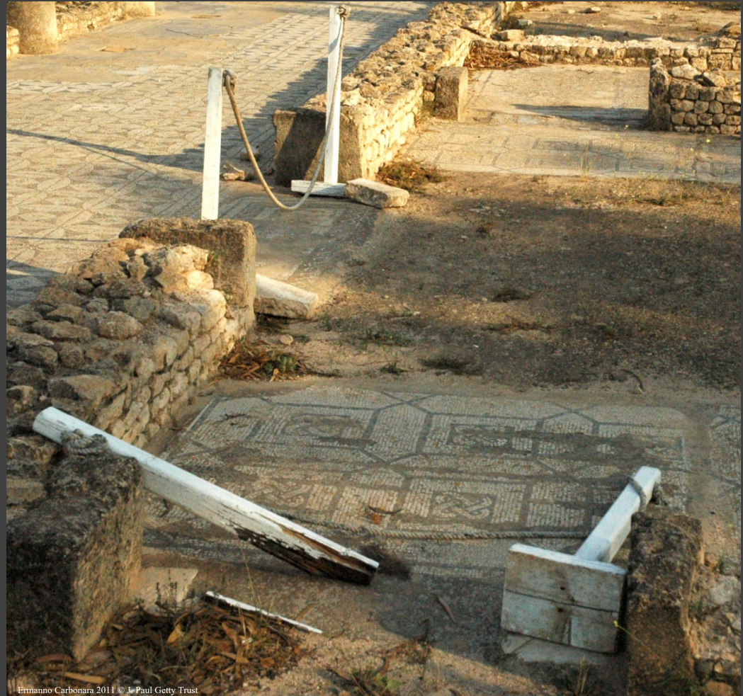
Damaged access barrier
