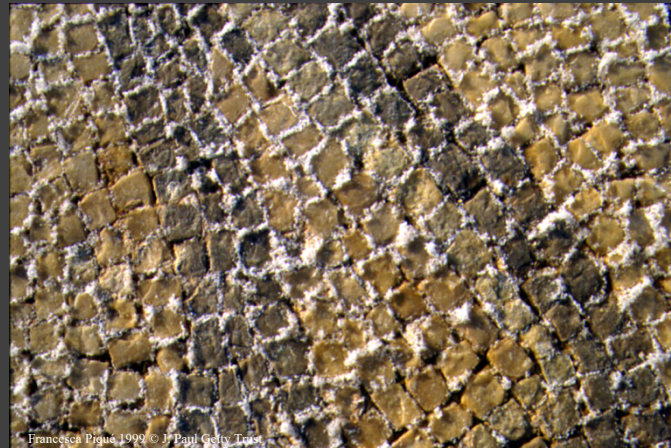
Efflorescence
