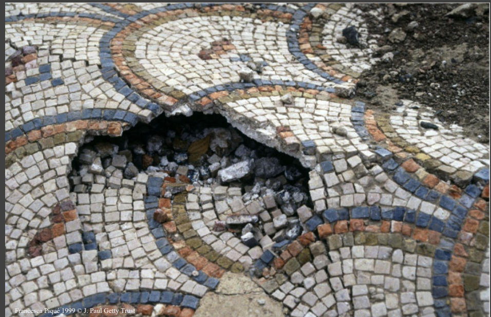
Bulges, Detachments, Cracks, Lacunae, Detached Tesserae
