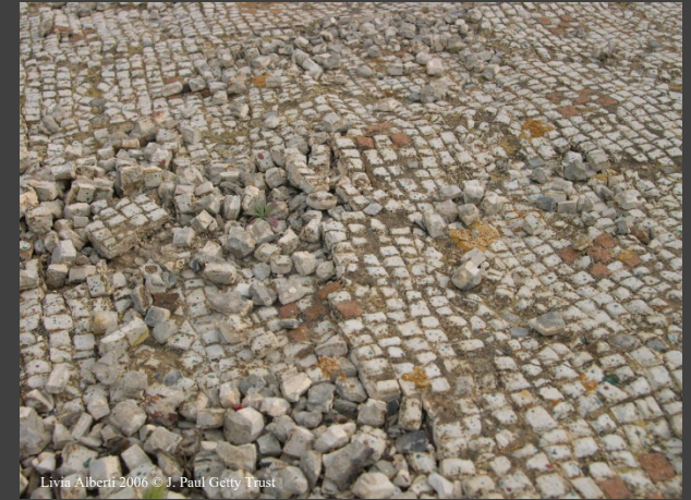
Bulges, Detachments, Cracks, Lacunae, Detached Tesserae
