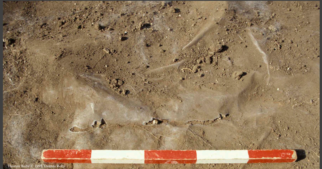
Deteriorated separation membranes
