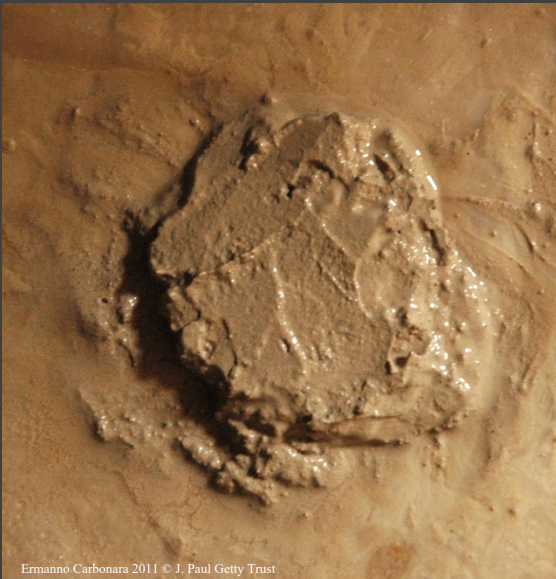
Mortar with too much water
