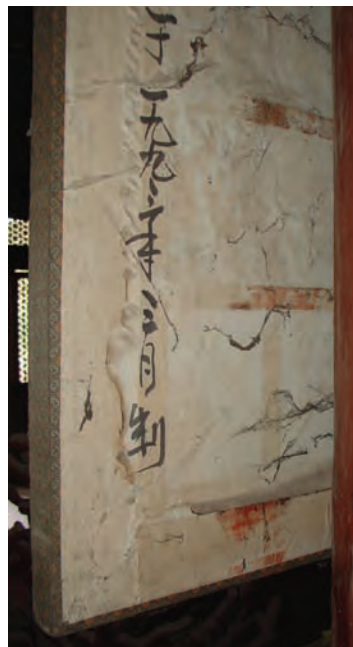
东侧楹联背面下方显示内部木质骨架的粘接剂污垢和1993年进行重新裱画的工匠名字。 Lower back of east couplet showing adhesive staining on interior wooden frame and the names of the craftsmen who carried out the reframing in 1993.
