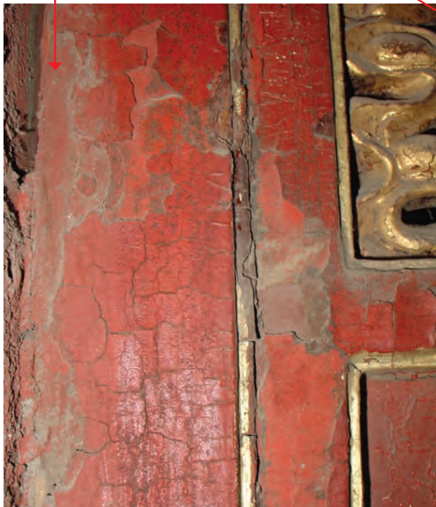
栏杆的状况。有两层红漆，底色是无光泽红漆，上层是光亮的红漆。 Condition of the balustrades. Note two layers of red paint including a lower matte red and an upper shiny red paint.
