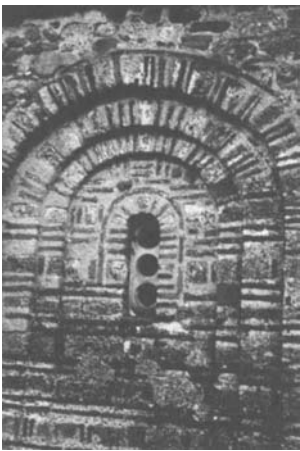
Figure 3.5 St. Nikita: north facade window.
