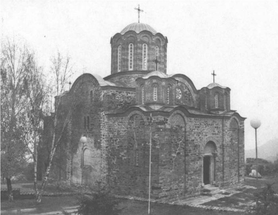
Figure 2.4 Quincunx church, St. Bogorodica, Matejče: north and west facades.
