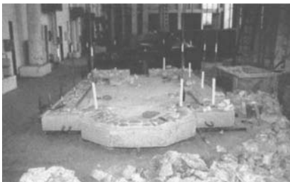
Figure 4.4 Model foundation during construction.
