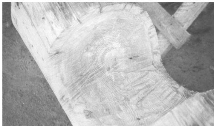
Figure 2 Joint cut in a 200-year-old log of European redwood in the Kenozero National Park. Note the minimal outer sapwood zone and the close, evenly spaced growth rings in the heartwood. Photo by Brian Ridout.
