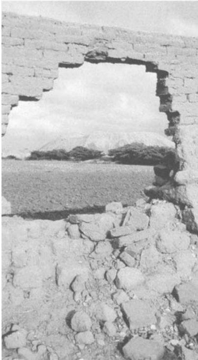
Figure 6 Deterioration and loss of construction materials in the perimeter wall. Photo by Carolina Castellanos.
