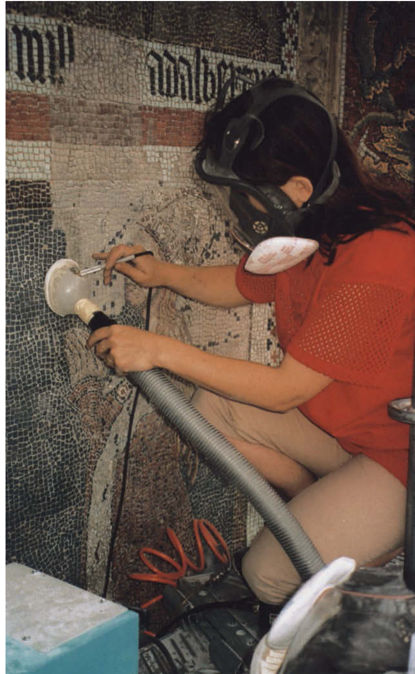
FIGURE 2 Removal of corrosion using a micro-abrasive device with crushed glass particles. Photo: D. Stulik.
