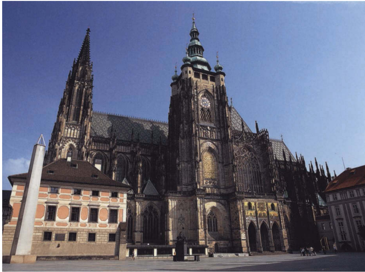
FIGURE 2 The south facade of St. Vitus Cathedral; the Last Judgment mosaic is seen over the south portal.
