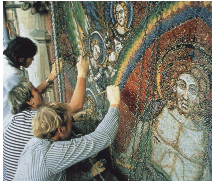
FIGURE 4 Conservation team applying the coating on the mosaic's central panel. Photo: E. Bescher.
