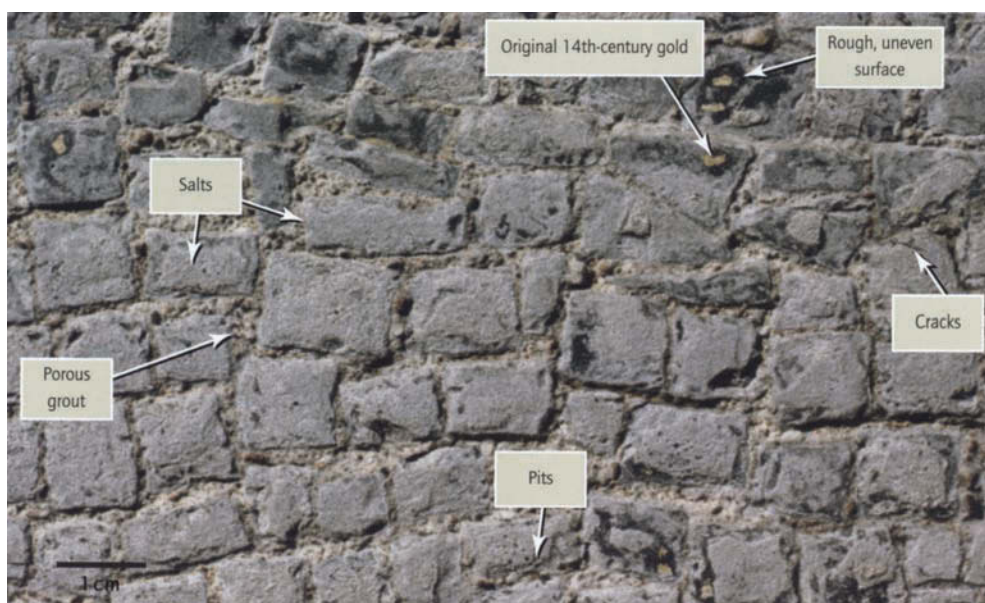
FIGURE 2 Photograph of a section of the mosaic before treatment, illustrating the complexity of the problem.
