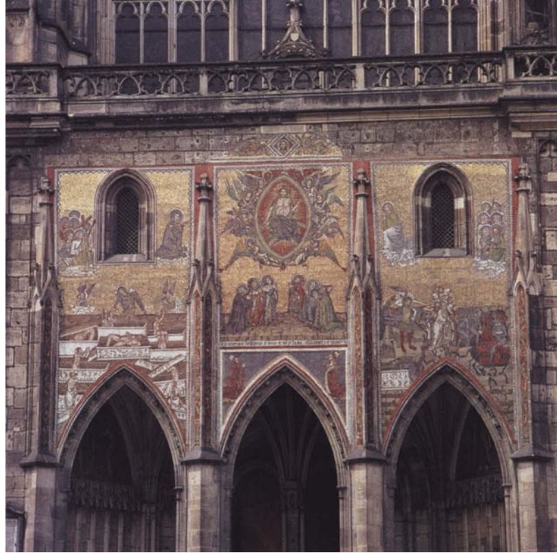
FIGURE 3 The mosaic in 1992, covered with a corrosion layer, at the beginning of the project. Photo: D. Stulik.
