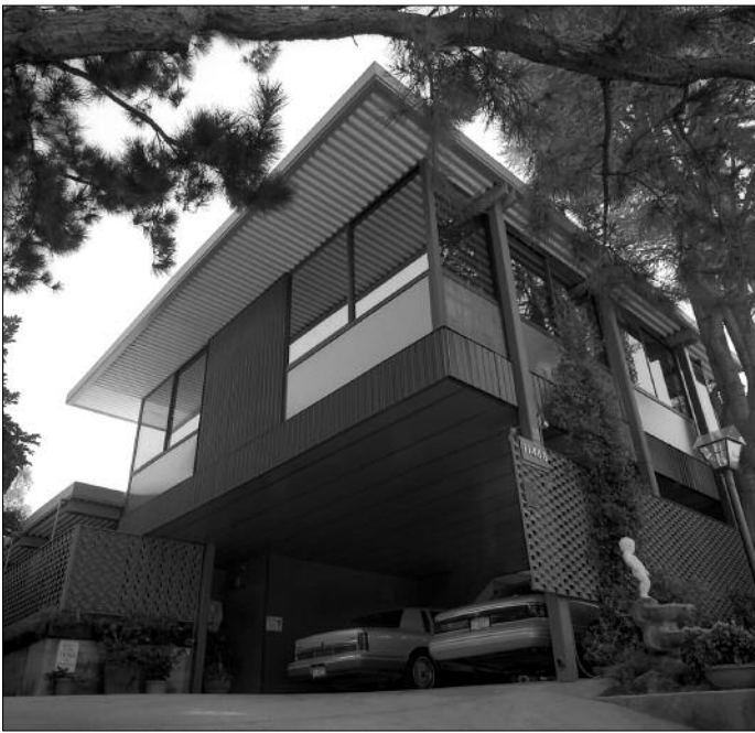
The single-family homes that have been designated as Los Angeles Historic-Cultural Monuments represent a wide variety of architectural styles and historical periods. Top: This house in Granada Hills was built in the late nineteenth century and was declared a Historic-Cultural Monument in 1996. Above: This Studio City home, built in 1964, was declared a Historic-Cultural Monument in 1997. As Historic-Cultural Monuments, both of these homes may qualify for historic preservation incentives. Photographs by John C. Lewis.
