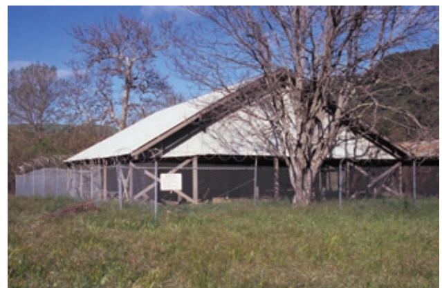
FIGURE 8 Las Cruces Adobe covered by a wood shelter that protects the ruins. Photo: Gail Ostergren.
