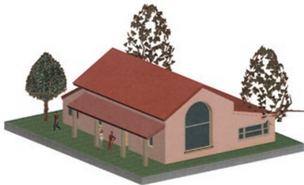
FIGURE 3 Casa de la Torre seen from the northeast corner. The retrofit included anchoring the adobe walls into the upper roof on all sides of the building; center core rods were also placed in the two walls that are visible.
