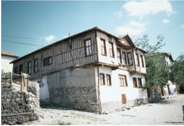
FIGURE 5 Himiş structure in Ayas, Turkey. The ground floor is constructed of stone and used for utility or domestic animals rather than for human habitation.
