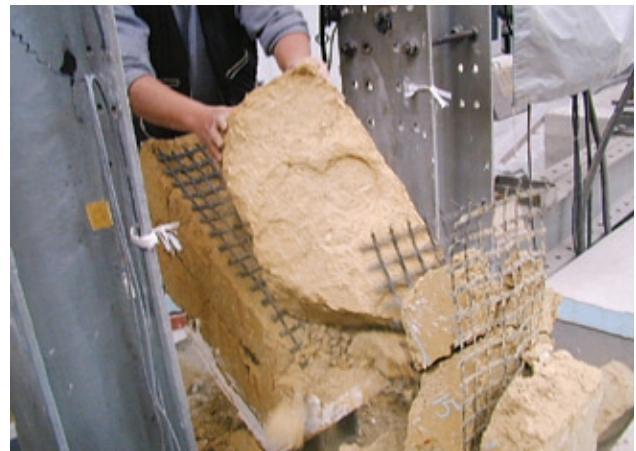
FIGURE 15 Horizontal joints in an earthen wall sample and their response to lateral forces.
