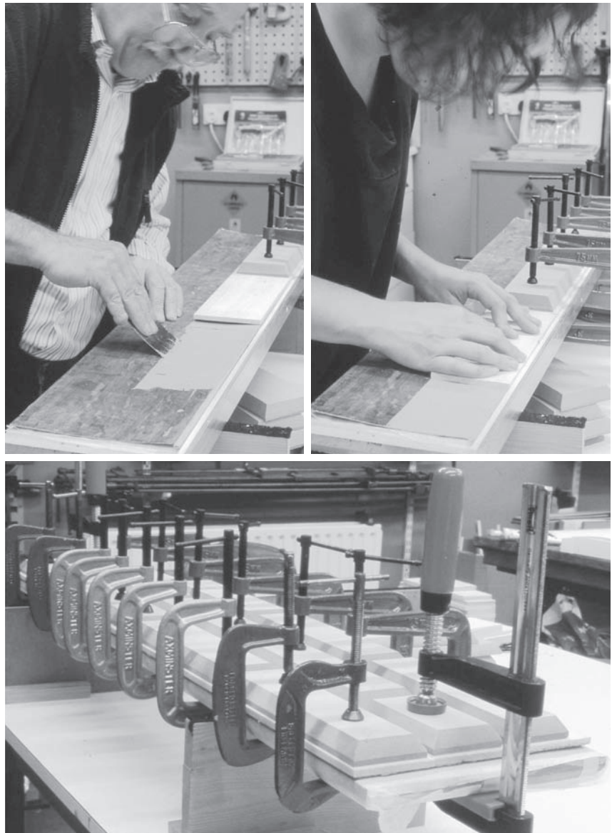
Figure 6 Application of the Araldite AV/HV1253 and balsa pieces. Photos: © Hamilton Kerr Institute. Fitzwilliam Museum, Cambridge.
