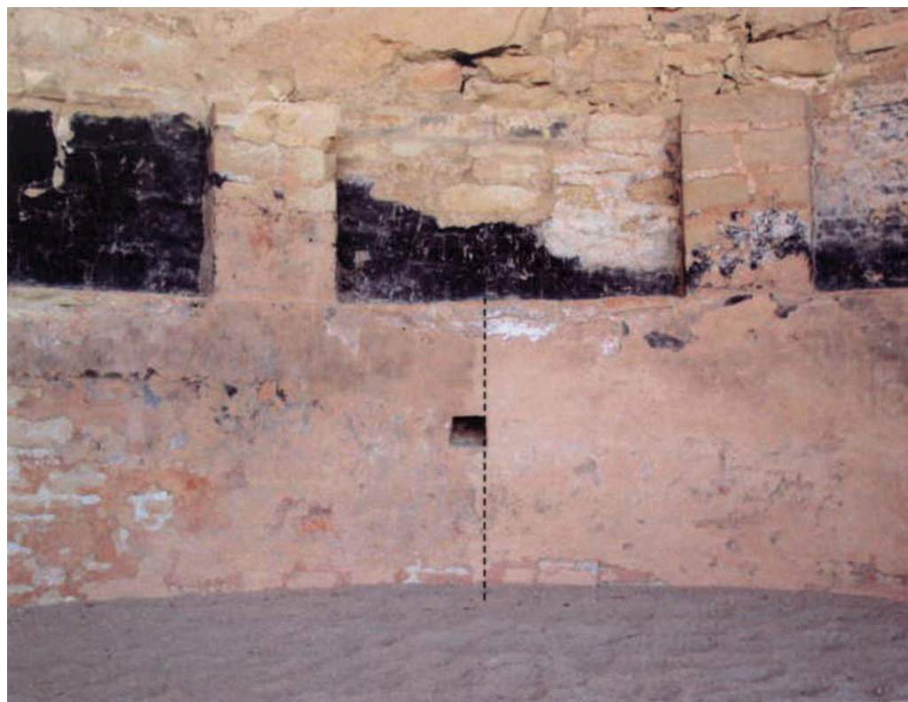
FIGURE 6 Coupled with the placement of Kiva Q, the symmetrical bichromatic application of plasters (indicated by the dotted black line) probably shows the integration of two social units becoming one. This building may have been the gathering space for dual societies.
