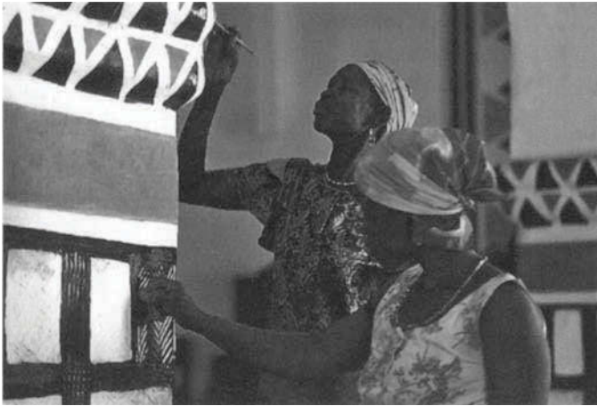
FIGURE 6 Sirigu women restoring the columns. Photo: Gisèle Taxil, CRA Terre-EAG, 2003.
