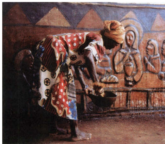
FIGURE 5 New scene at the entrance of the cathedral. This woman is using a vegetal broom to apply dawa-dawa , a local varnish. Photo: Gisèle Taxil, CRA Terre-EAG, 2002.
