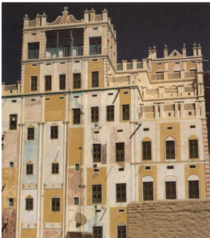
FIGURE 5 Exterior lime plaster and painted decorations require frequent renewal, as in this example of a Bugshan family palace in Khailah, in the left branch of Wadi Do’an.
