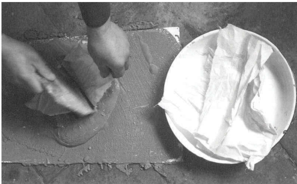
FIGURE 6 Yong'an Temple. A conservator is chopping the hemp paper into the fill mixture. Photo: Jun Zheng, 2000.
