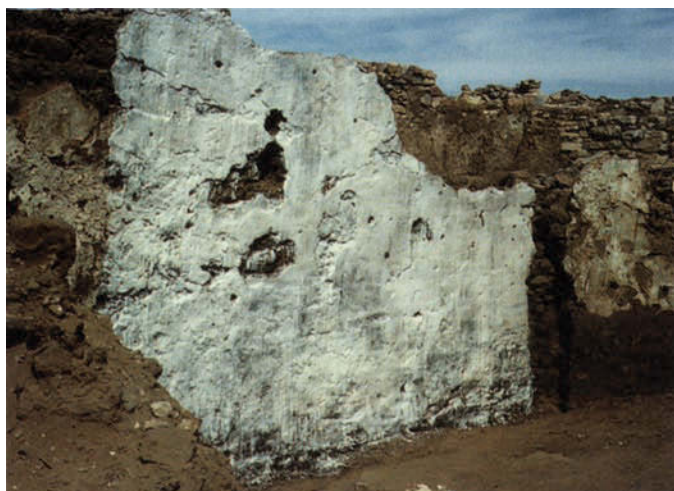
FIGURE 4 The section of wall painting to be removed has been consolidated and received its first coat of cyclododecane (February 2003). Gauze bandage was incorporated into the second, facing layer of CDD to fill in or cover the missing areas. Courtesy of the Egypt Exploration Society.
