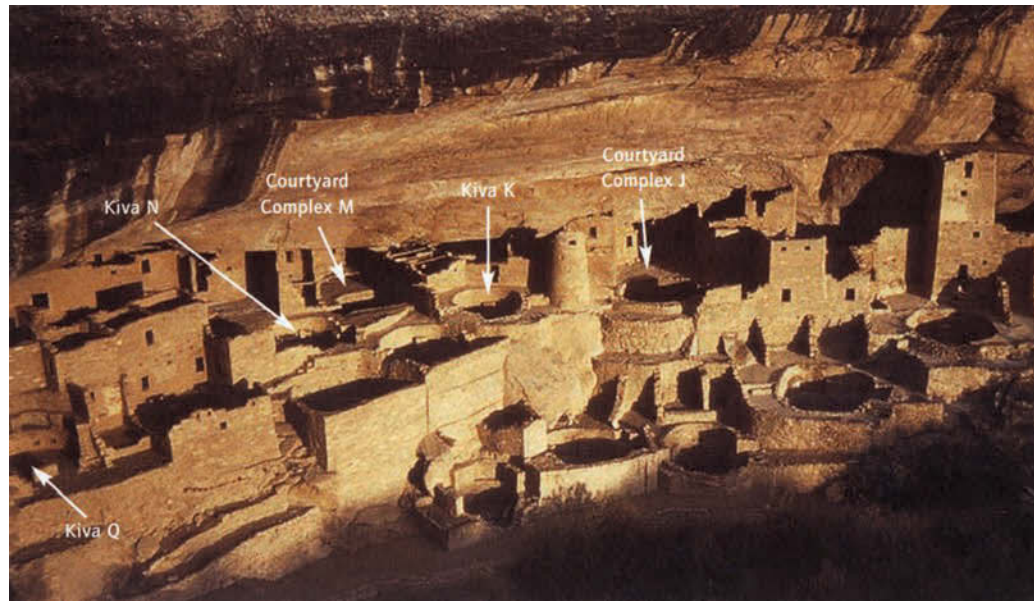
FIGURE 1 This overview photograph of Cliff Palace shows the village's architectural complexity. Circular structures below grade are kivas.
