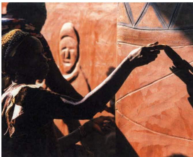
FIGURE 4 New scene designed at the entrance of the cathedral. Designs are incised on the still-wet surface with the edge of a flat stone. Photo: Gisèle Taxil, CRA Terre-EAG, 2002.
