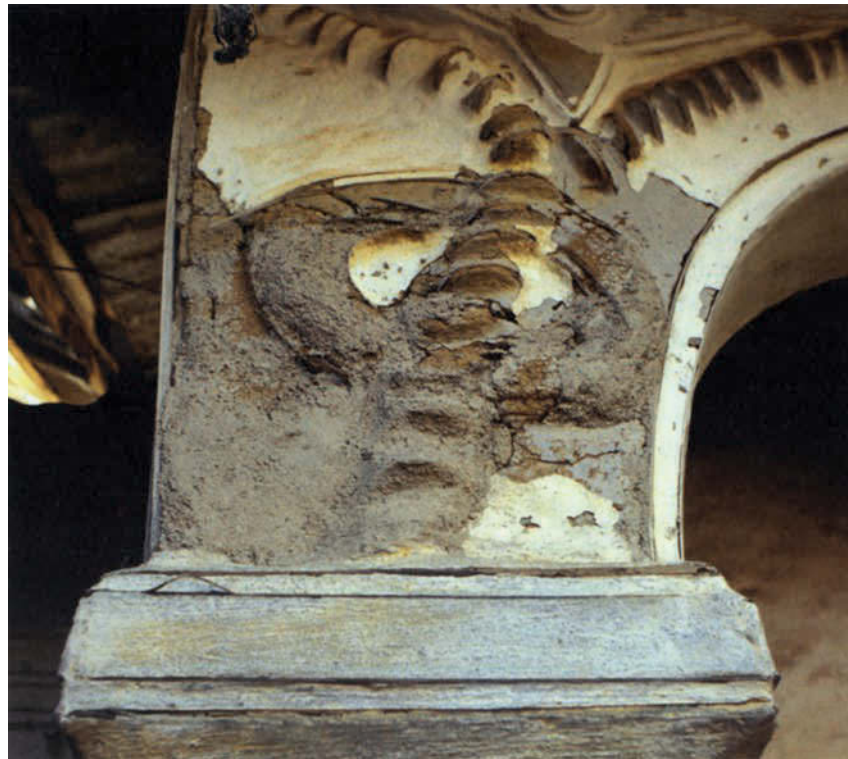
FIGURE 4 White decoration patched with cement (Asawase shrine). Photo: Sébastien Moriset, CRATerre-EAG.
