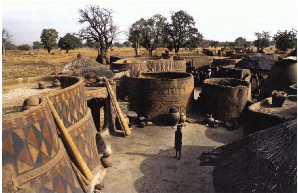
FIGURE 1 View of the courtyard and the dwellings of a traditional compound in northern Ghana. Photo: Thierry Joffroy, CRA Terre-EAG, 1997.
