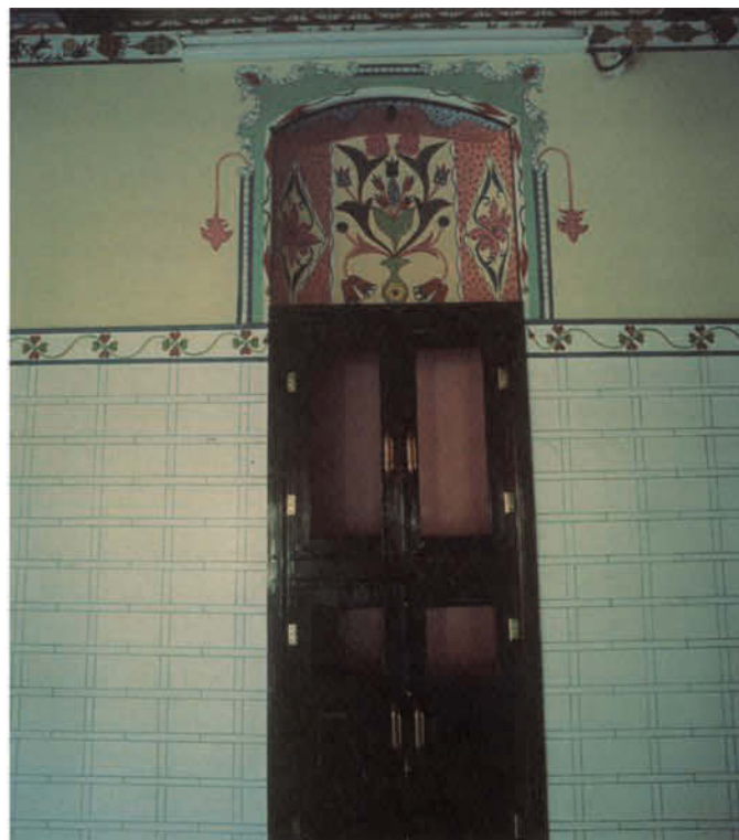
FIGURE 6 Malas , a form of highly burnished lime plaster, is a labor-intensive interior finish. In this contemporary example from the ba-Zaraah house in Khoreiba, Wadi Do’an, the malas has been scored to resemble ceramic tiles.
