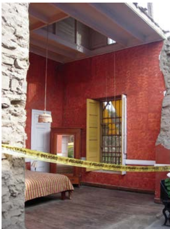
FIGURE 4.30 Out-of-plane of adobe wall failure due to lack of proper wall-roof connections. Main estate house, Hacienda San José, Cañete, as seen in October 2007.
