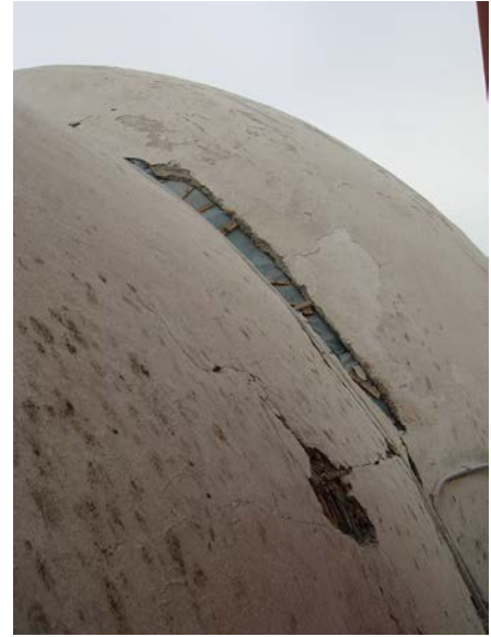
FIGURE 4.29 Detail of plaster detachment on dome at the Church of Chilca, in Cañete, as seen in October 2007.
