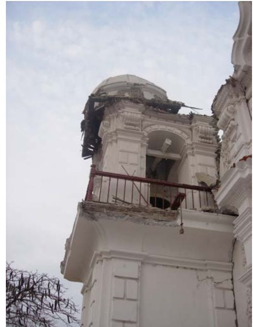
FIGURE 4.8 Detail showing shift of church tower dome at the Estate Church of San José, Cañete, as it appeared in October 2007.
