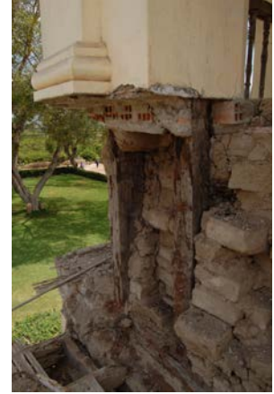
FIGURE 4.39 Detail showing the mixture of building materials used at the Hacienda Arona and Montalván in Cañete, as photographed in October 2007.
