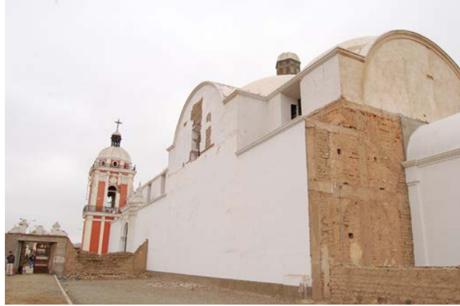
FIGURE 4.38 Detail showing the mixture of building materials used at the Church of Chilca, as photographed in October 2007.
