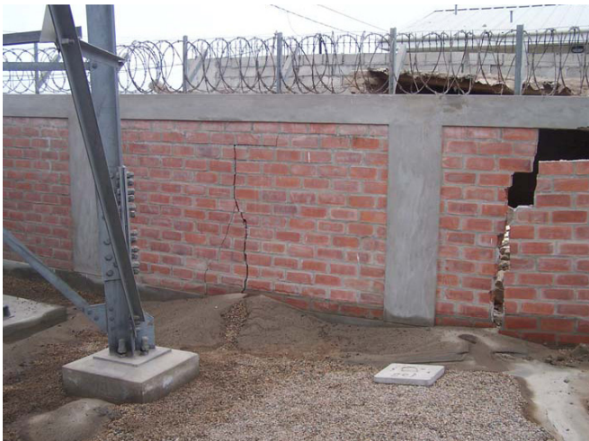
FIGURE 2.18 Liquefaction at a site in Tambo de Mora. Image: Courtesy Jorge Alva Hurtado.
