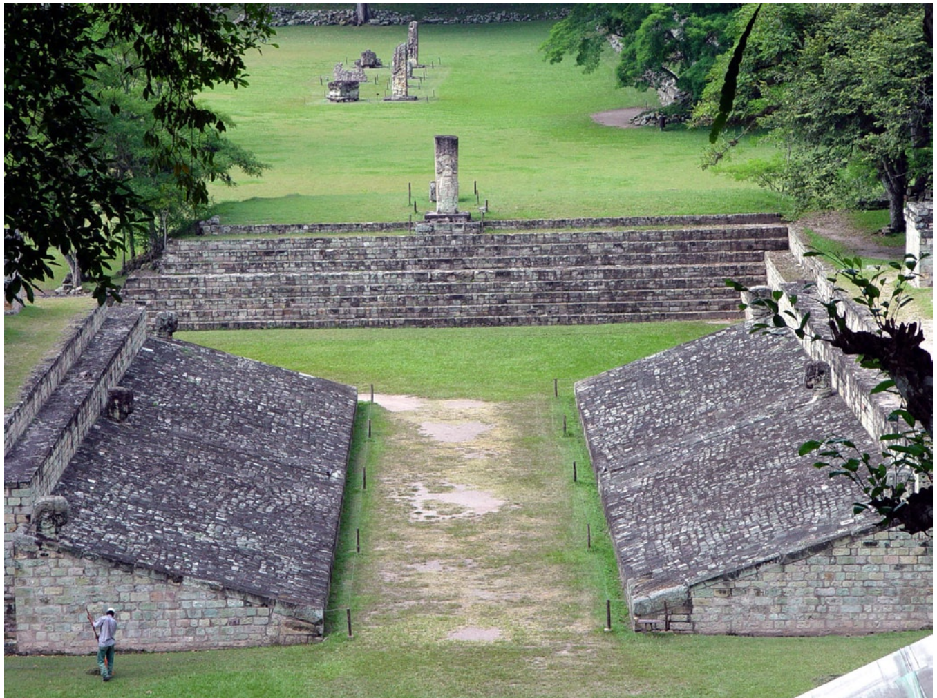
Figure 81 The present condition of the Ballcourt, showing a black patina on the horizontal surfaces and its absence on vertical surfaces.
