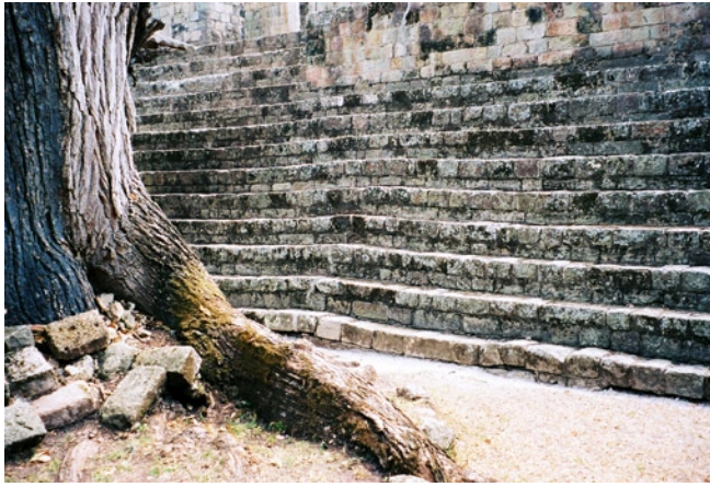
Figure 91 View of the stone steps of Structure 9, showing deformation from tree roots.
