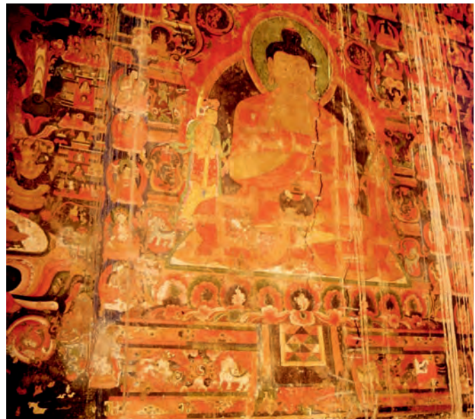
FIGURE 2 Section of the Chamba Lakhang's northeast wall, with a deep structural crack running down the center. The crack has been “stitched” with mesh strips (white patches) along its length.
