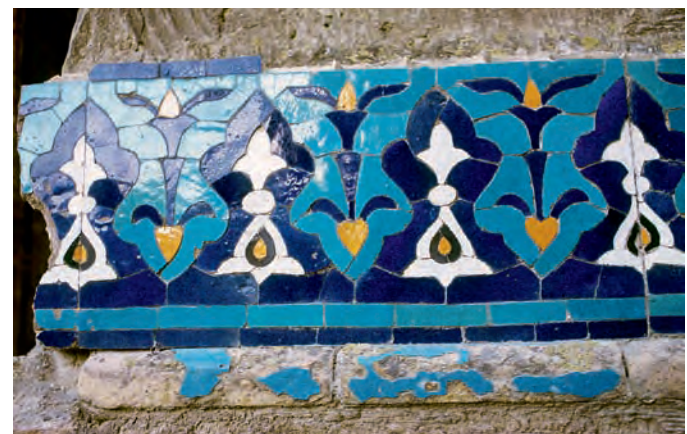
FIGURE 1 Tiles in yellow, white, a lapis lazuli or cobalt blue, and a turquoise or copper green from the Bibi Khanom mosque, sixteenth century. Tiles were glazed as large square tiles and then cut and ground to fit a flower-patterned frieze, using a Persian mosaic style of tile decoration.
