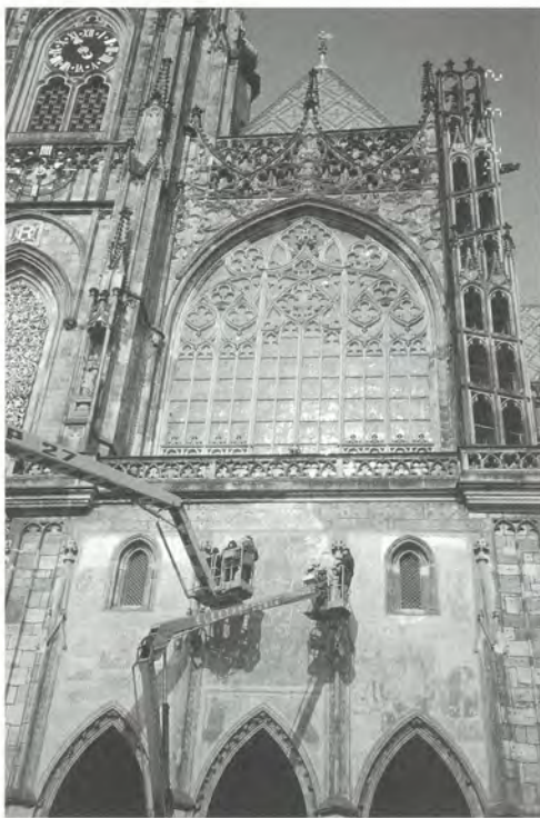
Top: A detail of The Last Judgment mosaic depicting the face of Christ. An opaque layer of corrosion products covers the glass mosaic's surface. Photo: Dusan Stulik. Bottom: Using a cherry picker, conservators assess the mosaic's condition while a television crew documents their work. Photo: Neville Agnew.
