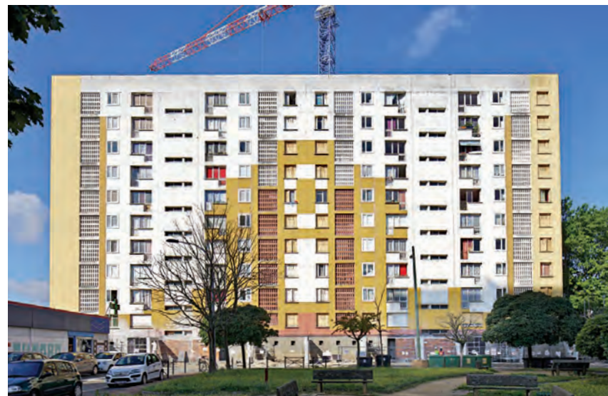
Cité du Grand Parc social housing, Bordeaux, France , before (left) and after (right) renovation by the firm of Lacaton and Vassal in 2016. Once demolition of this 1960s public housing complex was ruled out, Lacaton and Vassal reimagined three 10- to 15-story housing towers to give tenants more space and light, upgraded facilities, and improved energy efficiency. Using prefabricated materials, 530 units were rehabilitated without displacing residents. Although not conservation per se, the project demonstrates a sustainable approach that retains use and social values while reducing waste and meeting demands for carbon reduction in construction. Photos: ©Philippe Ruault-Photographer.
