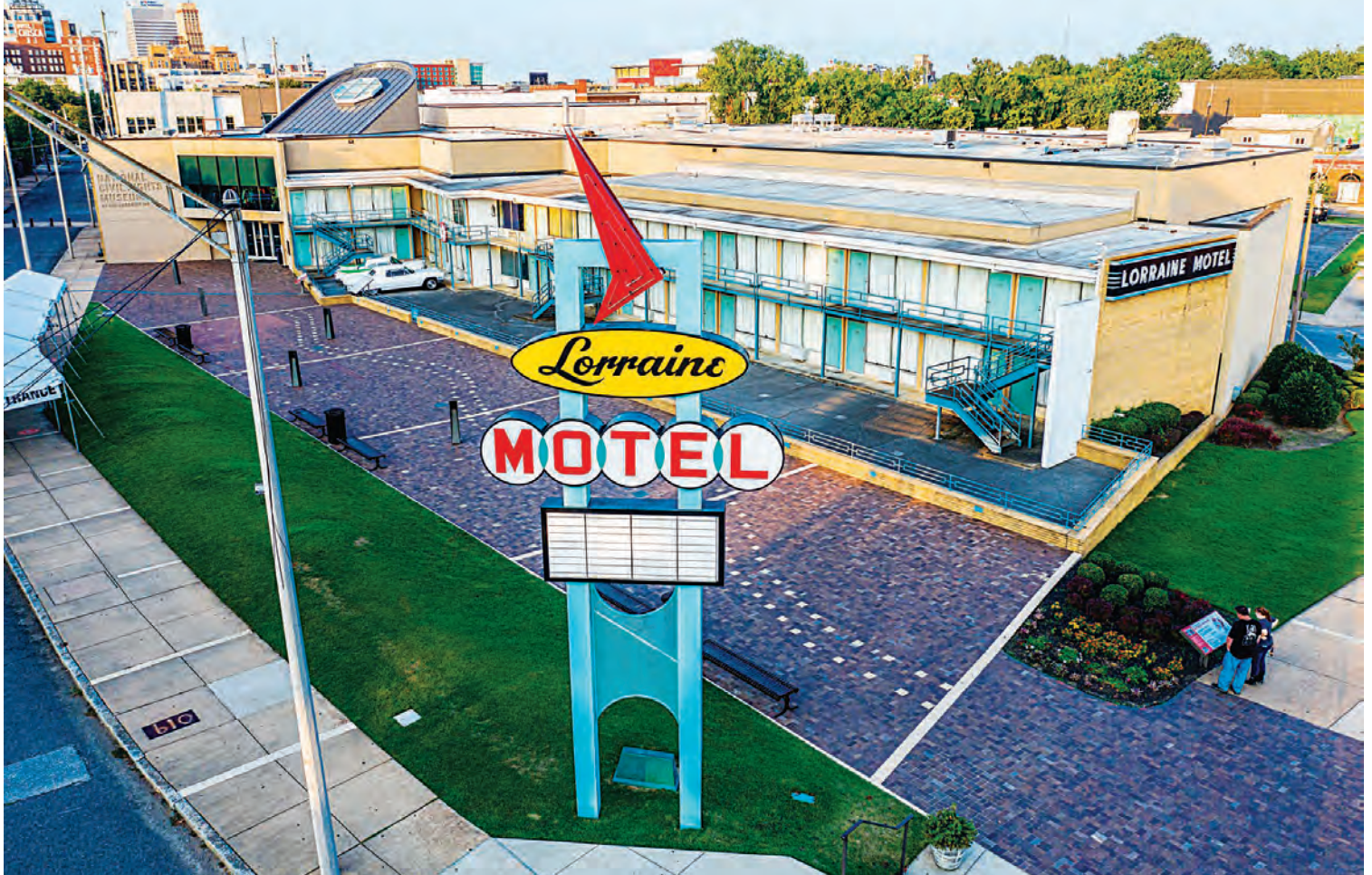
Lorraine Motel, Memphis, Tennessee. This example of everyday modernism is recognized for its role in the US Civil Rights Movement and is part of the International Coalition of Sites of Conscience. Built and owned by African Americans, the motel was safe lodging for Black travelers during segregation. In April 1968 civil rights leader Dr. Martin Luther King Jr. was assassinated while standing on its balcony. Following its 1988 closure, the building became the centerpiece of the National Civil Rights Museum, which opened in 1991. Photo: Madeleine Jettre / Alamy Stock.
