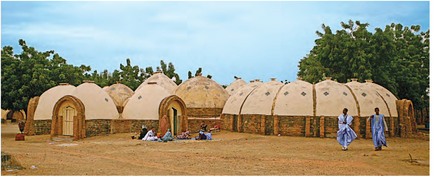
Kaédi Regional Hospital extension, Kaédi, Mauritania , designed by Fabrizio Carola and Birahim Niang and completed in 1992. To expand a conventional concrete-framed hospital building, the architects developed a low-cost approach utilizing local materials and labor. The resulting series of passively cooled and naturally lit mud-brick domes uses African concepts of modernity to meet contemporary needs. Photo: Alexis Doucet. Licensed under the Creative Commons Attribution-Share Alike 3.0 Unported license.
