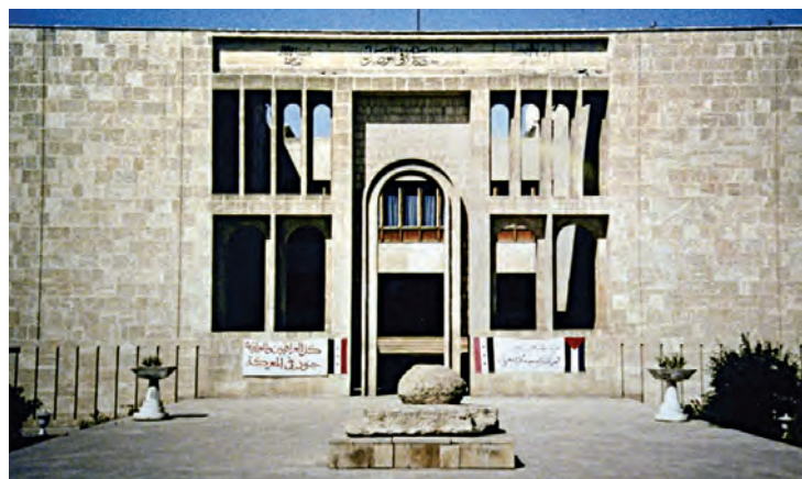
The Mosul Museum in Iraq in the early 1980s . Designed by Iraqi architect Mohamed Makiya, and opened in the mid-1970s, the building is a national modern heritage landmark. An international project is working to rehabilitate the building in the wake of its destruction by ISIS in 2015. Image in the public domain.
