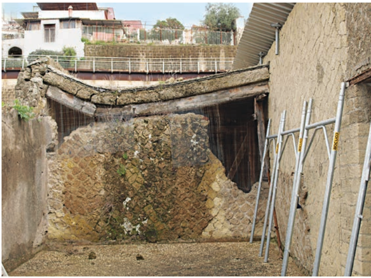
Left: A collapsed concrete slab at the House of the Bicentenary, from the 1939 period. This is how it appeared in March 2018. Photo: Paola Pesaresi/Herculaneum Conservation Project. Right: The same spot after the concrete slab was replaced with a new wooden structure, with work completed in late spring 2019. Photo: Di Lauro/Herculaneum Conservation Project.
