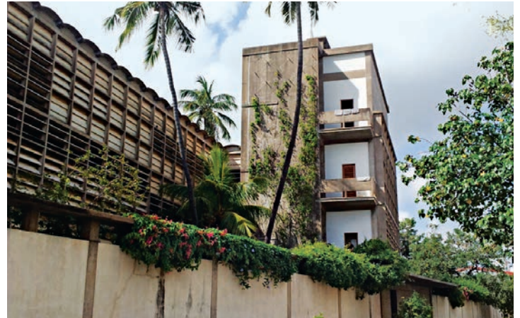
The Golconde, constructed between 1937 and 1942 in Pondicherry, India, and designed by Antonin Raymond and George Nakashima. Photo: Aleksandr Zykov, licensed under the Creative Commons Attribution-ShareAlike 2.0 Generic license.
