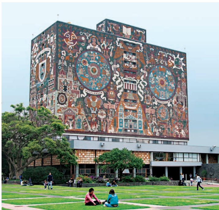
The Central Library of the National Autonomous University of Mexico. The building, designed by architect and artist Juan O’Gorman with architects Gustavo Saavedra and Juan Martínez de Velasco, opened in 1956 and includes O’Gorman’s mural, Representación histórica de la cultura , a splendid example of integrated art and architecture. Photo: Susan Macdonald, GCI.
