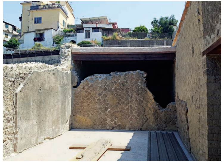
Left: A collapsed concrete slab at the House of the Bicentenary, from the 1939 period. This is how it appeared in March 2018. Photo: Paola Pesaresi/Herculaneum Conservation Project. Right: The same spot after the concrete slab was replaced with a new wooden structure, with work completed in late spring 2019. Photo: Di Lauro/Herculaneum Conservation Project.
