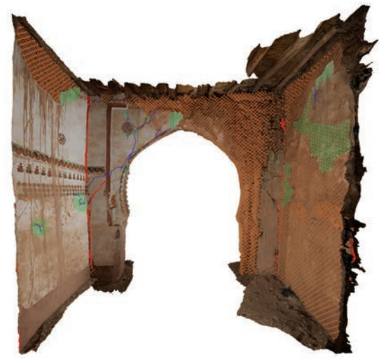
Two-dimensional condition maps of the interior decorative surfaces at Kasbah Taourirt, Ouarzazate, Morocco (left) converted into three-dimensional models to correlate interior conditions with structural problems (right). Images: Lori Wong and Samuel Whittaker, GCI.
