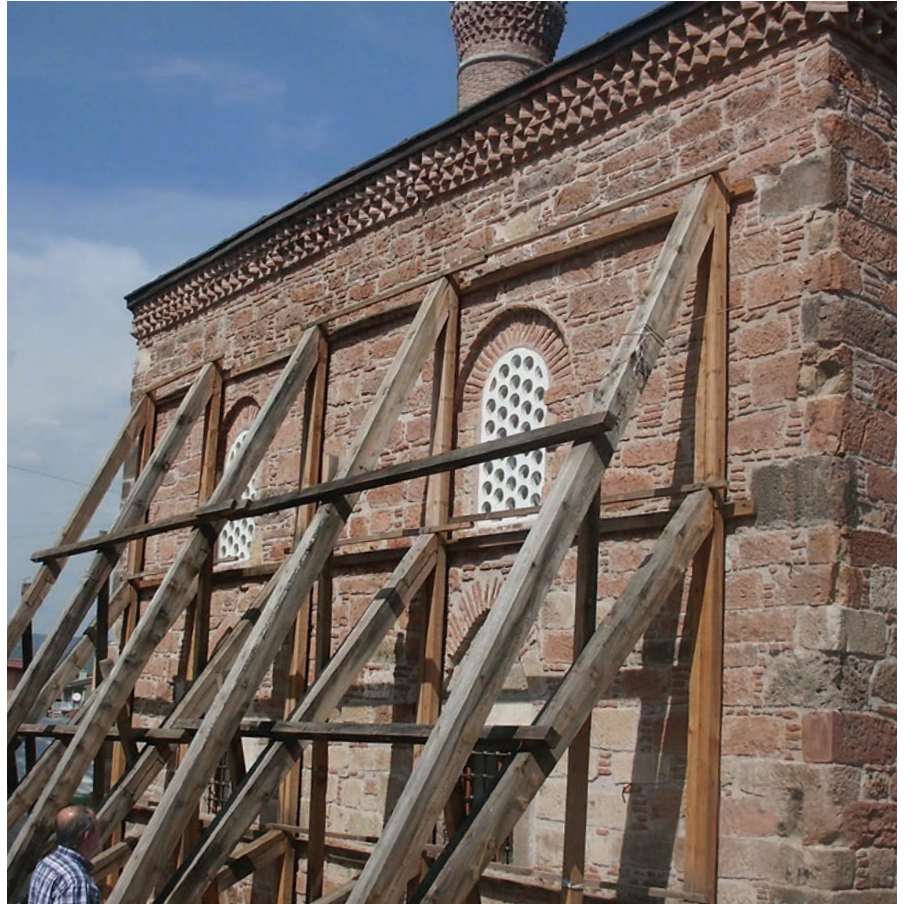
Emergency structural support for the Nasuh Ağa Camii (mosque) in Simav, Turkey, following a 2011 earthquake. Photo: Courtesy of the Republic of Turkey Ministry of Culture and Tourism, Cultural Assets Preservation, Regional Directorate Board of Kütahya.
