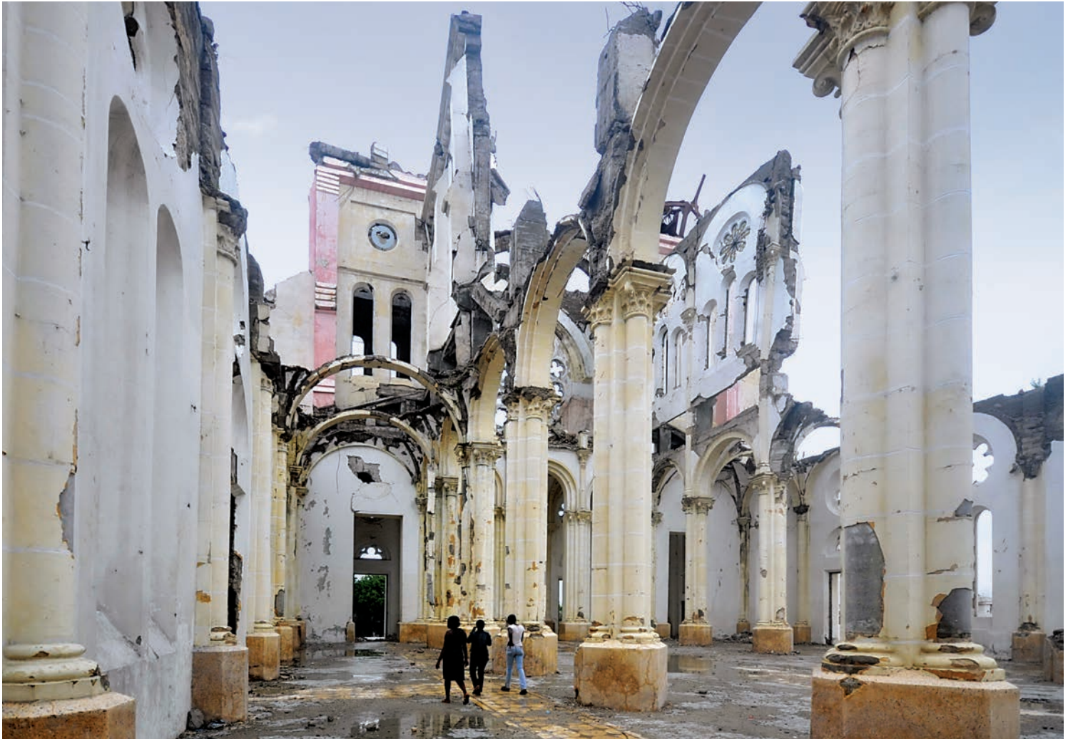
The reinforced concrete Cathedral of Our Lady of the Assumption (1884–1914), also known as the Port-au-Prince Cathedral. The cathedral was destroyed in the January 2010 Haiti earthquake. Photo: Stephen Kelley.
