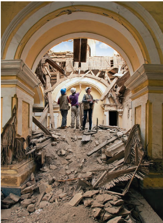
ON THE COVER A 2011 assessment of earthquake damage to Ica Cathedral in Peru, conducted as part of the GCI's Seismic Retrofitting Project. Photo: Scott S. Warren, for the GCI.
