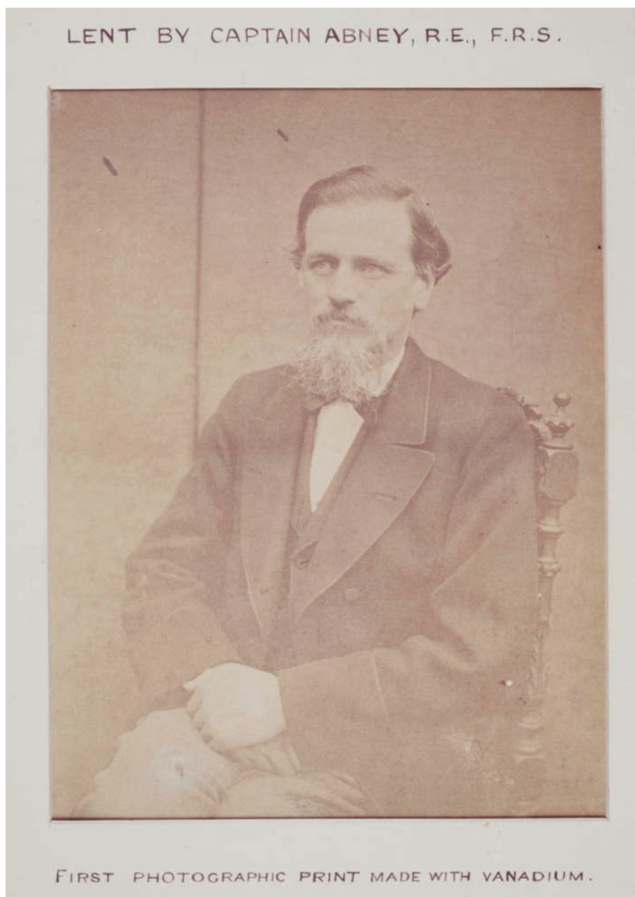
A print labeled "First Photographic Print Made with Vanadium." The GCI conducted XRF and FTIR analysis of the photograph—attributed to William de Wiveleslie Abney—and identified it as a salt print with no vanadium. Photo: Dusan Stulik, GCI.
