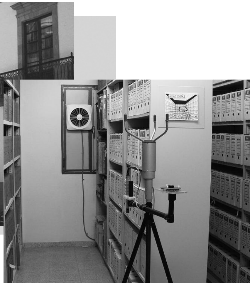
Above: The 19th-century building that houses the Historic Archive located in Tenerife's La Laguna historic district—a UNESCO World Heritage Site. Right: The climate control system installed in the archive as part of the GCI's Collections in Hot and Humid Environments project. In the foreground are monitoring sensors; at the rear is a window-mounted exhaust fan. Photos: Shin Maekawa.
