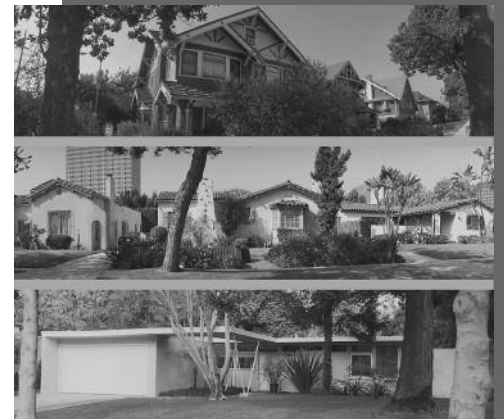
Incentives for the Preservation and Rehabilitation of Historic Homes in the City of Los Angeles
