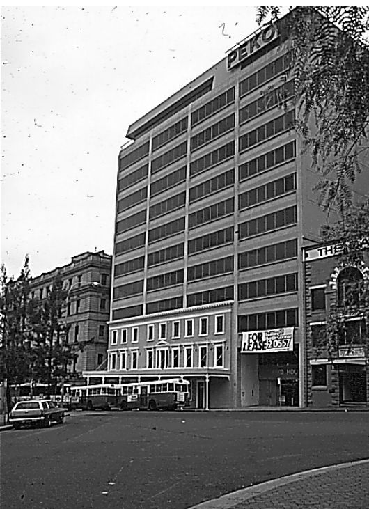
An example of facadism in Sydney, Australia. Preserving a historic facade while replacing the rest of the building with an unsympathetic modern construction destroys the continuity of a historic environment. Photo: Jukka Jokilehto.
