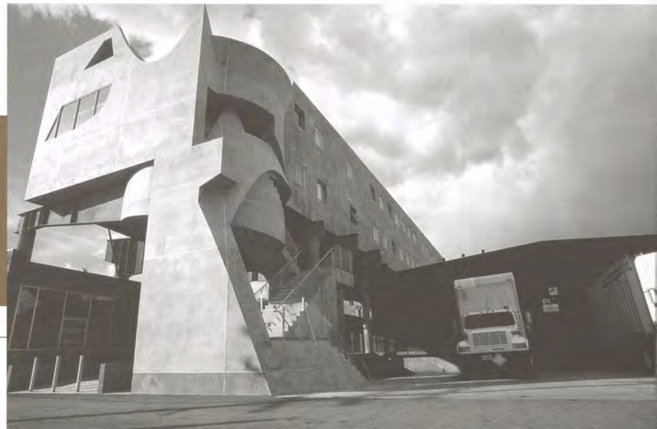
The Samitaur Building, leased by Kodak. The building, one of the early Smith-Moss projects, utilizes airspace above a private street, and has brought renewed economic activity to the surrounding, pre-existing warehouse structures. Photo: Eric Blanc.
