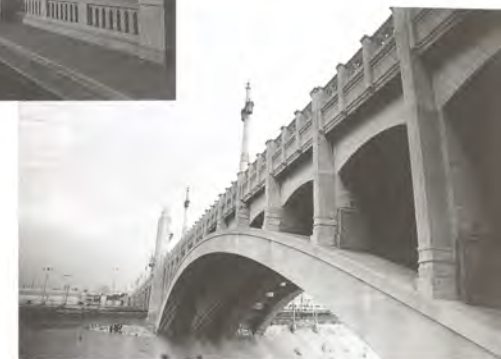
Below: A view of the Fourth Street Bridge. Photos: Gregg Gannon.
