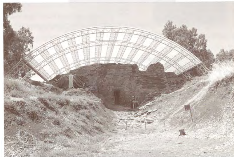
The Tel Dan gate in Israel. This 3,700-year-old mud brick gate is one of the earliest known examples of an arched structure. Discovered less than 20 years ago, the gate is now protected by the large shelter seen here. The GCI will be working with Israeli authorities to develop strategies for the gate's conservation, preservation, presentation, and maintenance. Photo: Lori Anglin.
