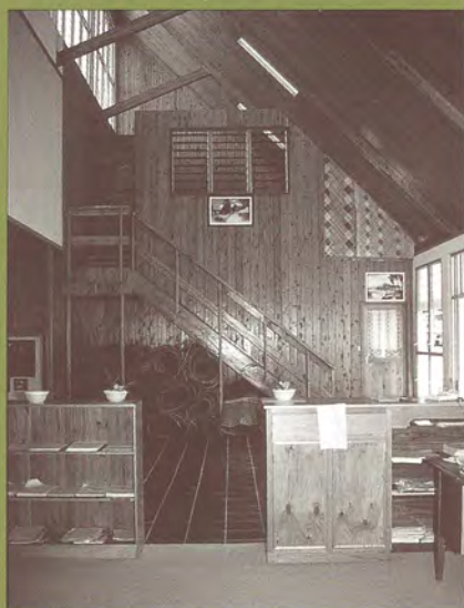
Exterior and interior views of the Kiribati Cultural Centre, which houses the National Museum of Kiribati, a Pacific Island State in Micronesia. The building's design permits air movement without mechanical ventilation. The louvered windows at ground level enable breezes from the sea—just 50 meters away—to pass through the building. The vents at the top of the building promote air movement through the stack effect (i.e., hot air rising). Photos: Colin Pearson.
