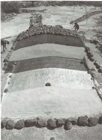
A cross section of the Laetoli trackway reburial stratigraphy, including layers of geotextiles. Photo: Angelyn Bass.
