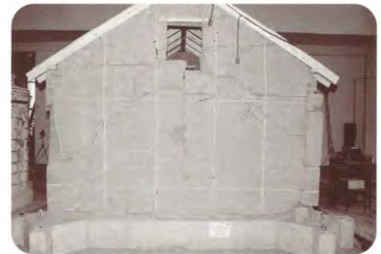
The gable end wall of a retrofitted tapanco adobe model after a test of equal intensity. Photos: William S. Ginell.
