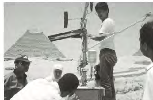
A GCI-designed environmental monitoring station being installed in 1990 on the Great Sphinx at the Giza Plateau. Photo: Neville Agnew.
